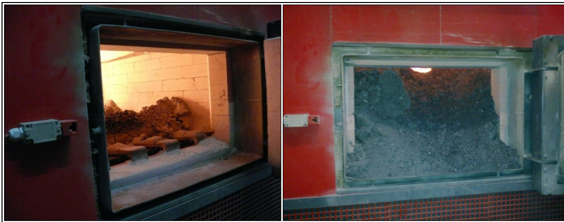
Figure 23 Boiler of the Marum biomass plant at the start of the test run and after approximately six hours when ash accumulation on the ash removal grate led to a shutdown.
